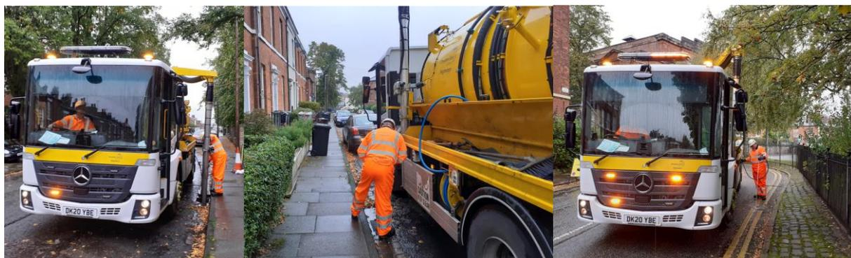
**Level 1** – Safe and serviceable: A scheduled programme of gully cleaning is undertaken across the road network to ensure that the collection of waste is removed so water can flow freely.
